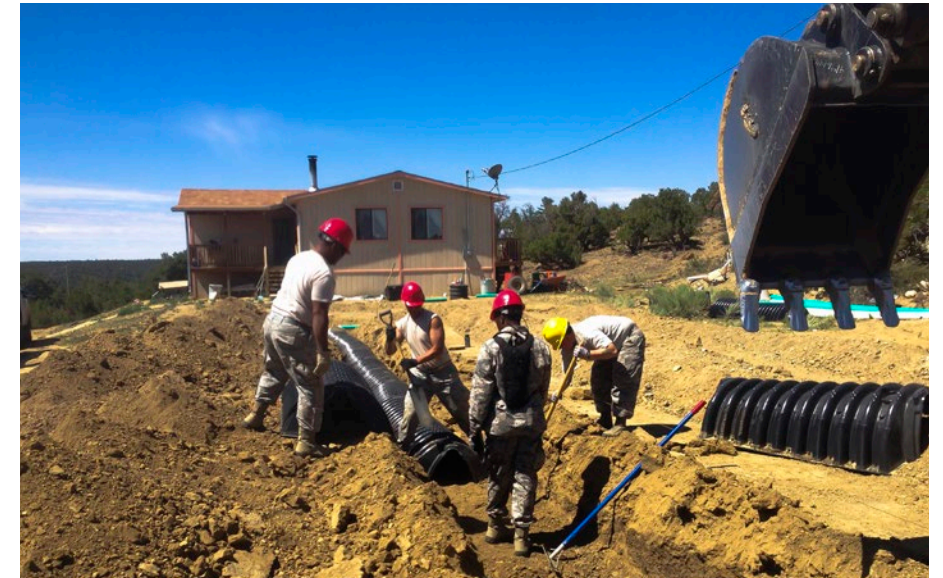
Four members of the 507th Civil Engineer Squadron install a new drain for an existing home on the Navajo Nation reservation in Gallup, N.M. in July. The team partnered with a local charity and constructed homes for impoverished Indians as part of Innovative Readiness Training. (U.S. Air Force photo/1st Lt. Christopher Yates)
